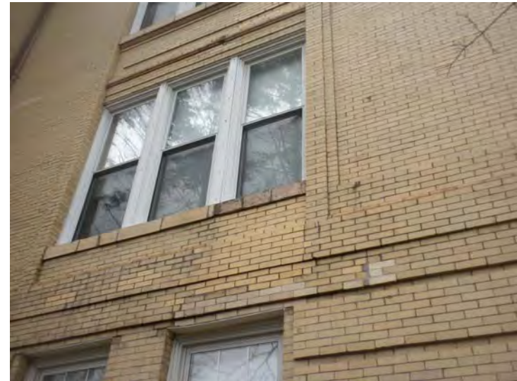
Minor mortar loss and evidence of past masonry repairs
