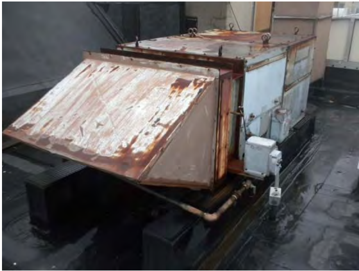
Roof-top unit. Abandoned in place
