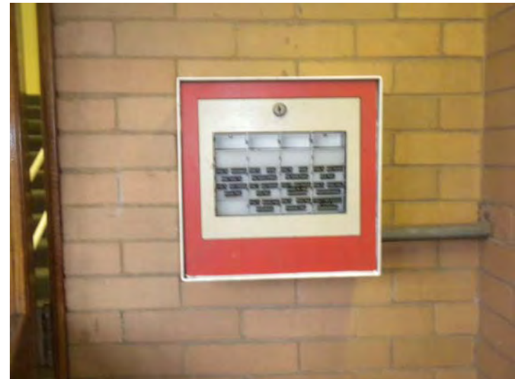
Fire alarm annunciator in the front vestibule
