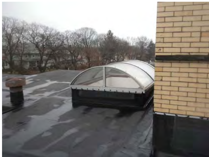
View of a dome type skylight
