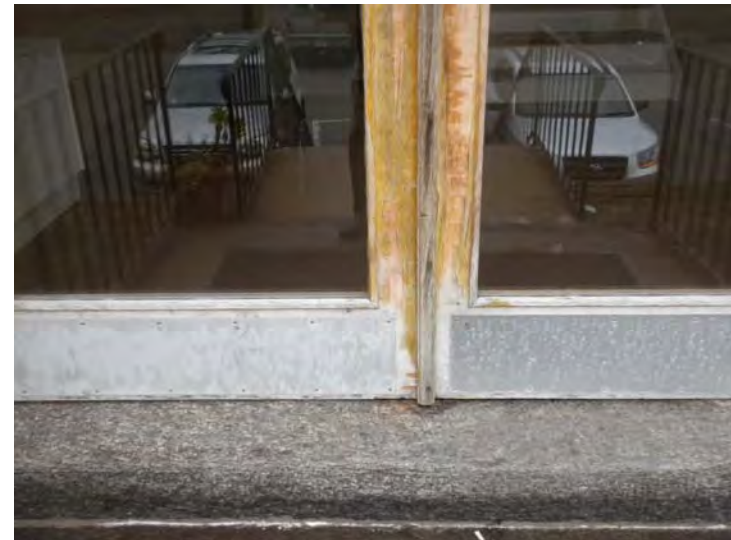
Example of age related wear to one of the wood entry doors
