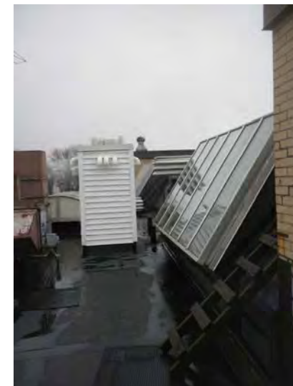
View of a panel type skylight
