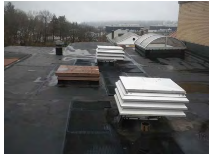
View of roof top exhaust fans
