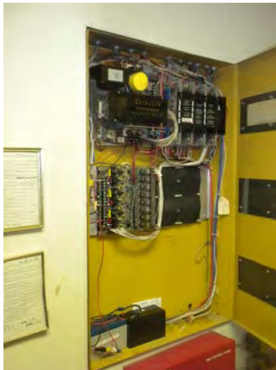
View of the fire alarm control panel
