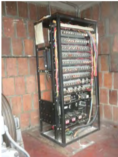
Open/close contact elevators controls
