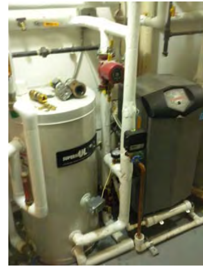
Each unit is served by a boiler providing heat and domestic hot water
